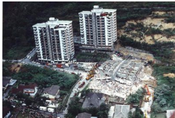
Fig. 1. The collapse of Highland Towers
