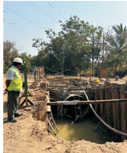
Fig. 11. Ongoing construction of electricity line
