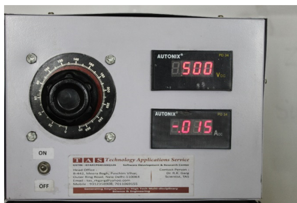
Fig. 4. High voltage DC power supply system
