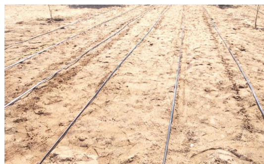
Fig. 2. Installation of drip laterals
