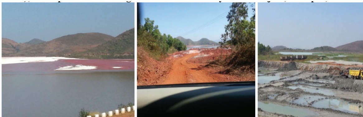
Photo 3. Red mud pond; Photo-4: Red mud used for road construction; Photo-5: Fly ash used for field preparation and road construction.
