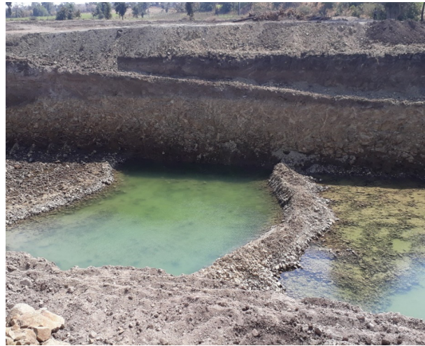
Fig. 1. Bunds dugout in the soil at Shirpur
