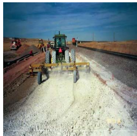
Fig. 3. Stabilization with Lime
