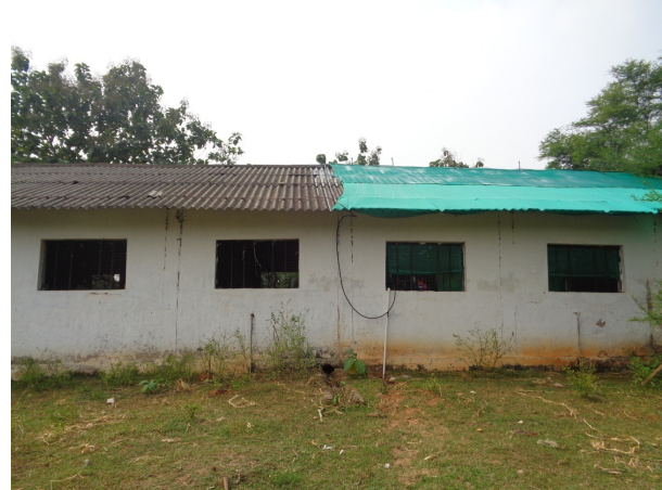
Fig. 1. Outside view of the normal asbestos shed and shed-net covered shed
