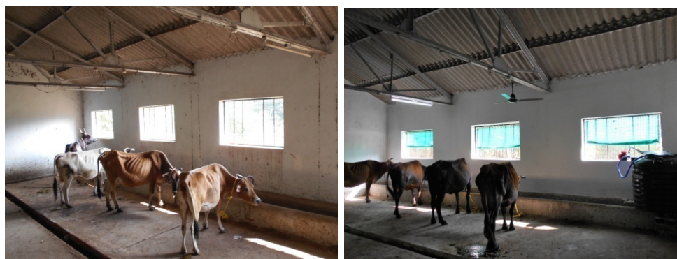
Fig. 2. Inside view of the normal asbestos shed and shed-net covered shed
