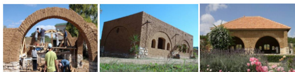
Fig. 5. Some achievements with adobe at the site of Sidi Amor - Tunisia
