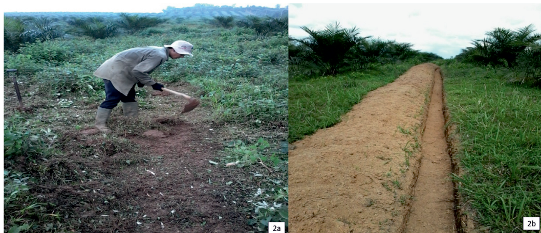
Fig. 2. Treatment plot of disposal ditch 2a under construction, finished drain ditch 2b. Every 2 rows of oil palm plants are treated with 1 drain ditch, the dimensions are: top width 50 cm, depth 50 cm, bottom width (bottom hole) 40 cm, and length 72 m.
